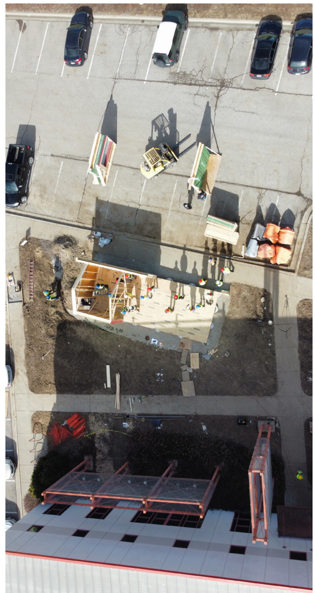
Haven Studio, aerial photograph of the construction site
